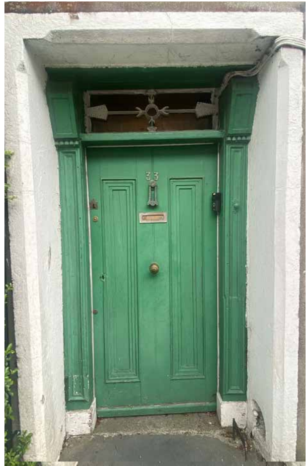
Figure 55 - Door and surround, Bridge Street
