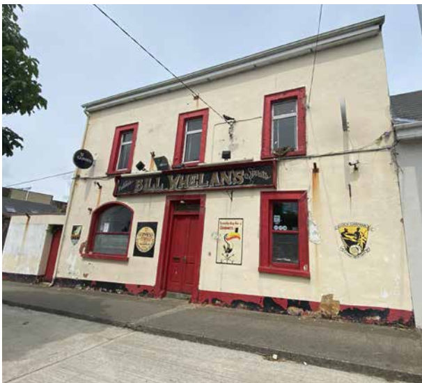
Figure 60 - Much altered historic pub, Irishtown
