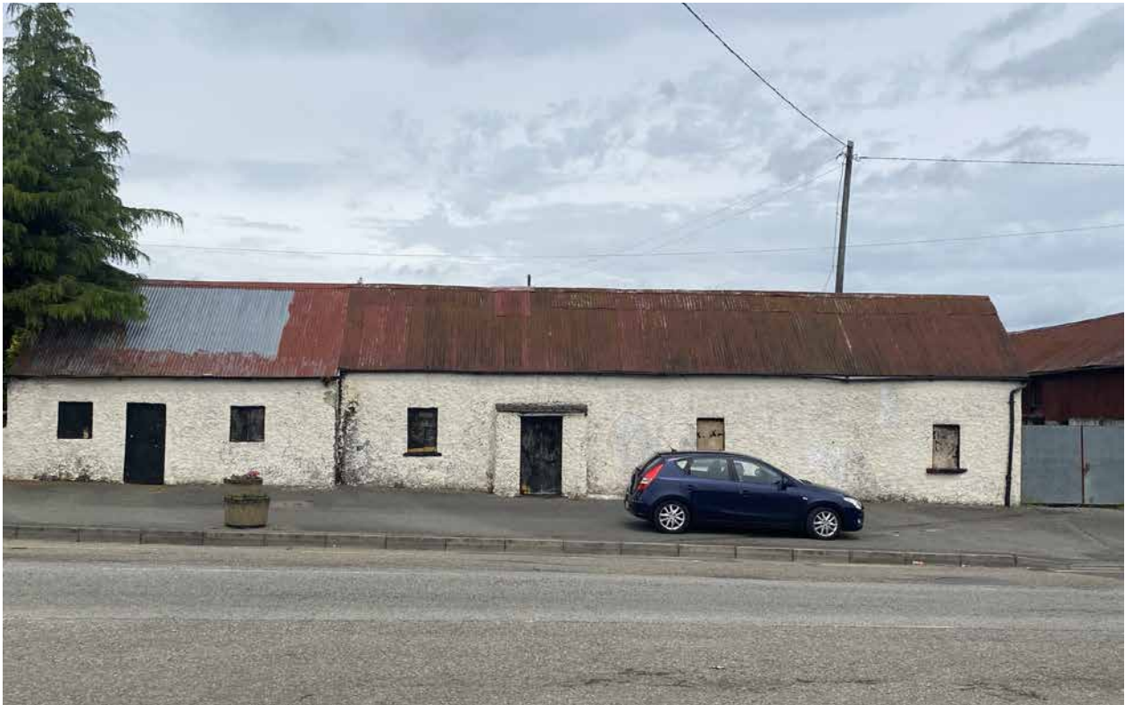
Figure 38 - Vacant historic cottages, Irishtown
