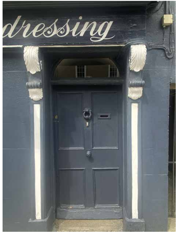
Figure 54 - Detail to historic shopfront
