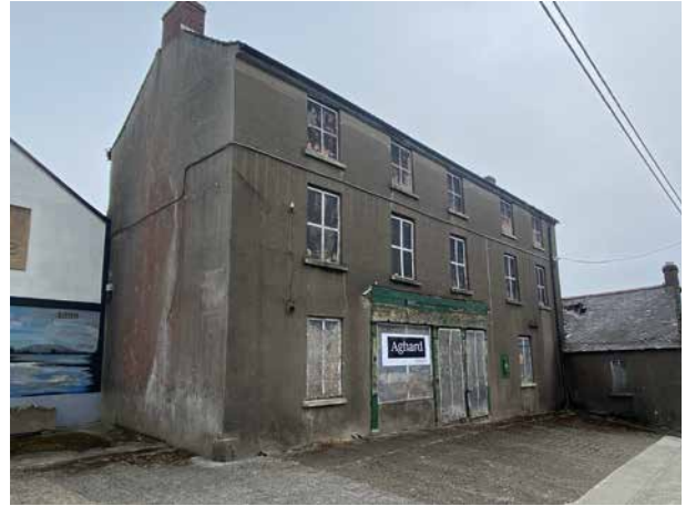
Figure 41 - Vacant building, Houghton Place
