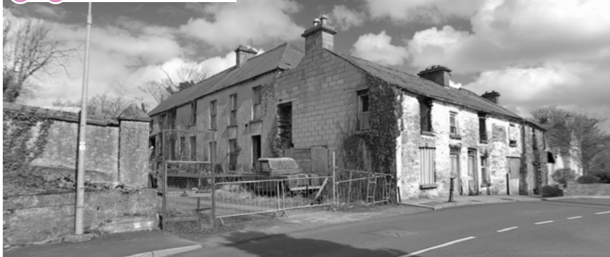
2 & 3 Existing heritage buildings.
