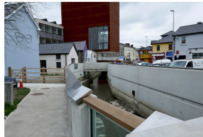
Caol Stream after flood defence works
