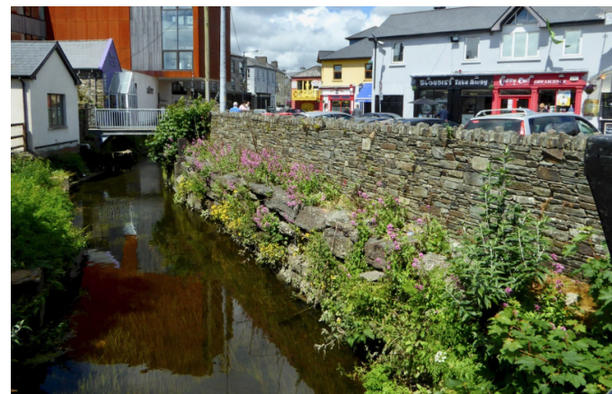
Caol Stream before flood defence works
