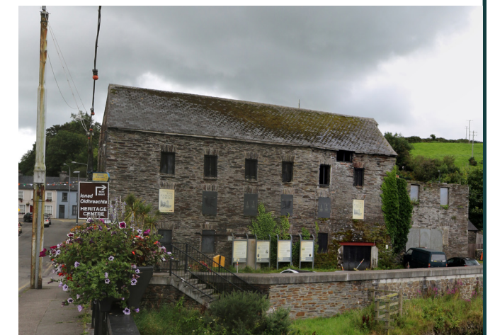
North Elevation of Steam Mill
