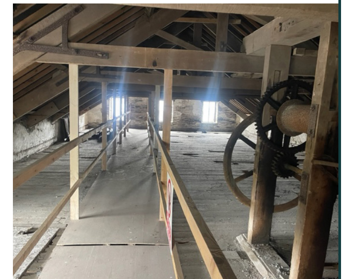
Interior of Steam Mill
