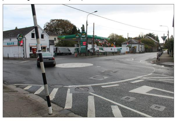
Figure 4.5 Bridge Street / Clara Bridge Mini-Roundabout (no crossings and narrow footpaths)
