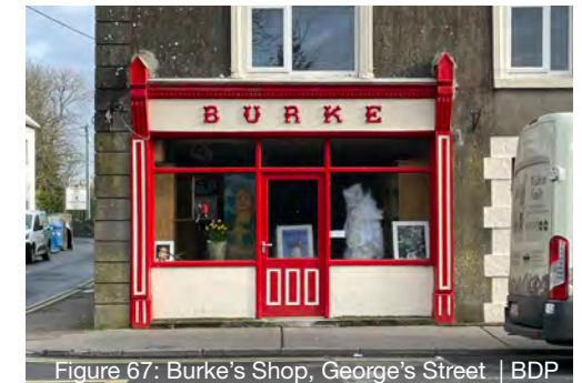
Figure 67: Burke's Shop, George's Street | BDP
