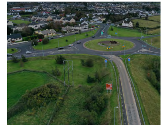
Figure 61: Roundabout at Junction 16 from the M18 Aerial View | Source: GCC
