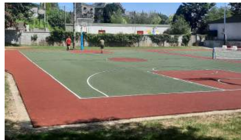
Thomastown Recreational facility
