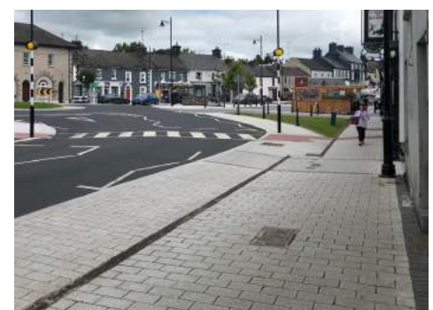
Project example - Virginia paving
