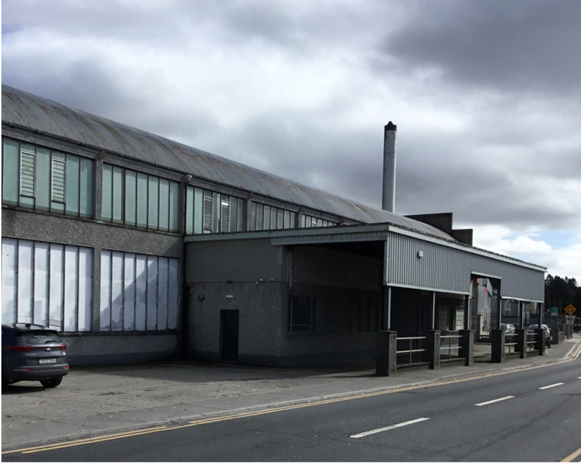
Figure 5-11: Former Pharmaceutical Factory Site (Antigen) on Lourdes Road.
