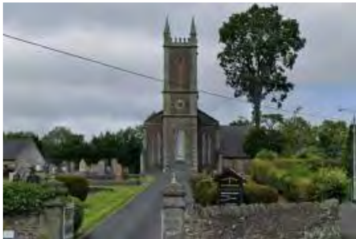
Figure 24 - Bailieborough Church Of Ireland - Current
