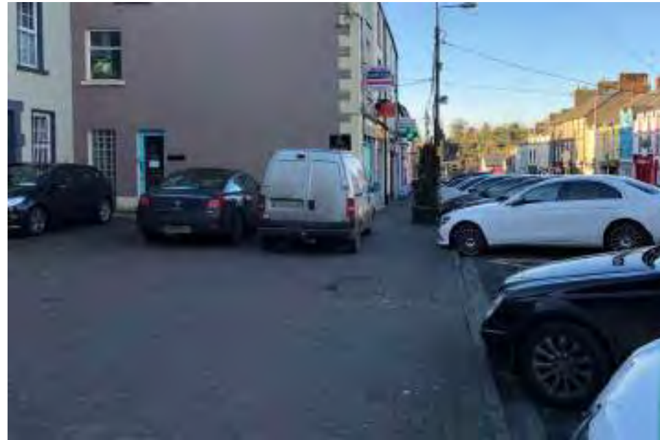
Bailieborough - existing: uneven paving littered with chewing gum and current design enables parked cars to overlap the kerb.
