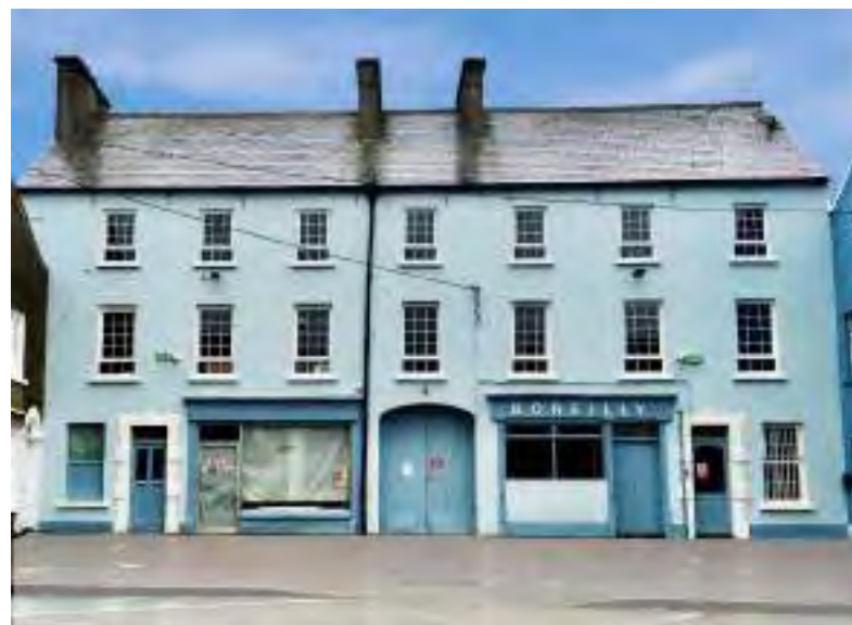
Figure 74 - Bailieborough Main Street - After Painting Scheme
