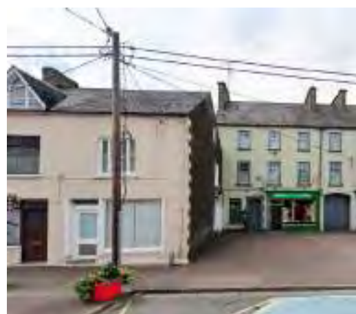
Figure 86 -Bailieborough Main Street - Existing overhead cables and Damaged Paving
