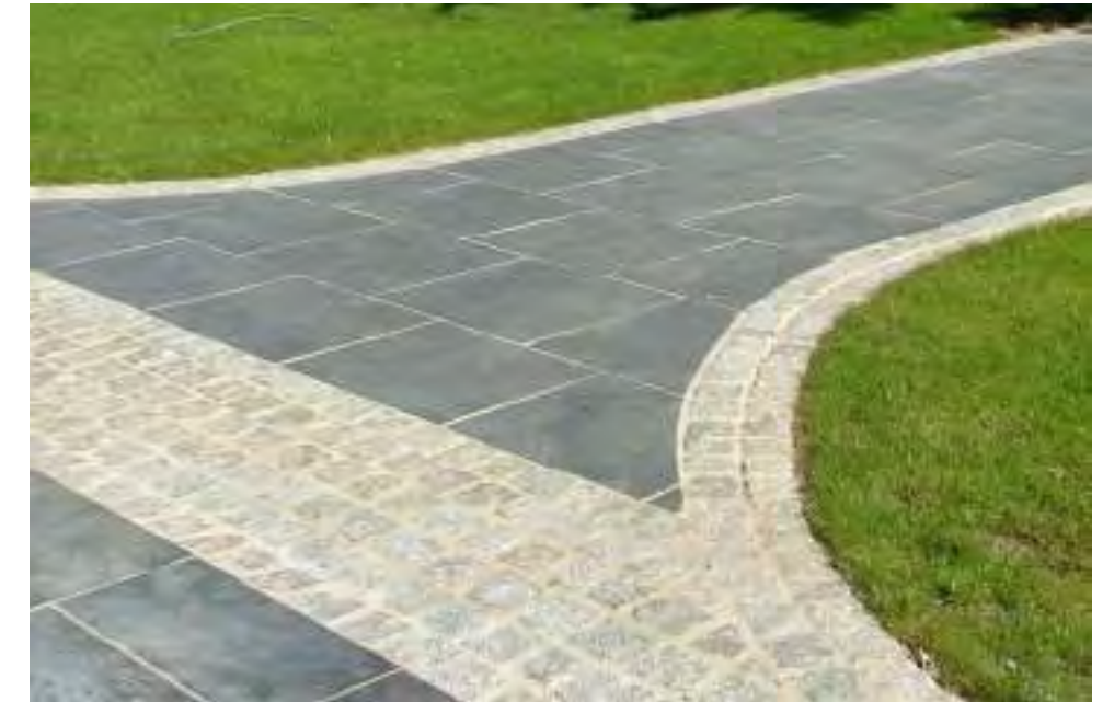
Proposed: use of local materials to create aesthetically pleasant and well designed pathways. Consider application of cobbles/textured grain to edges and thresholds.
