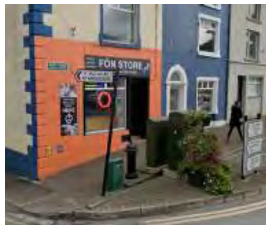
Figure 82 - Bailieborough Main Street - Signage, Utilities and Damaged Paving
