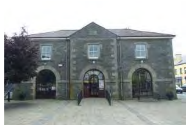
Figure 26 - Market House - Current
