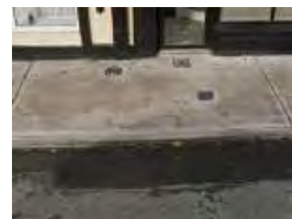
Figure 90 - Pavement at Barrack Street
