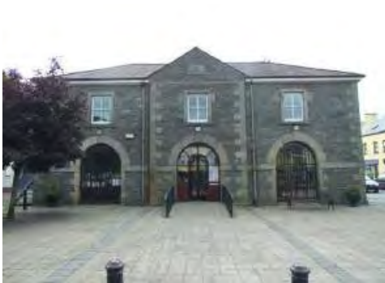
Figure 73 - Bailieborough Library After
