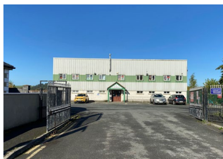
St Kevin's Community Centre, Main Street
