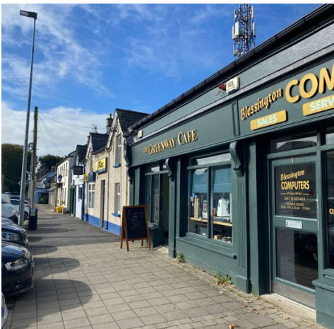
Generally wide stretches of footpath with examples of attractive shop fronts enriching the historic character of the town.
