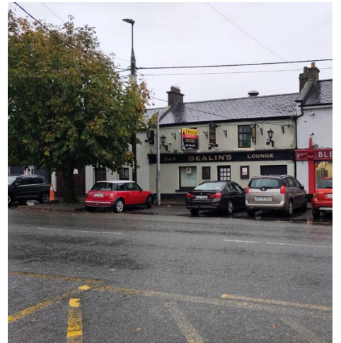
Overhead electrical cabling is a constraint to retention of existing street trees and planning for more.
