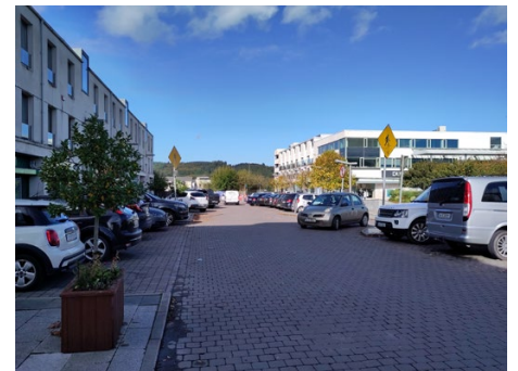
Opportunity Site 6 lies within the middle ground of the photograph - the hoardings of which provide a focal point for those driving along Newtown Square.
