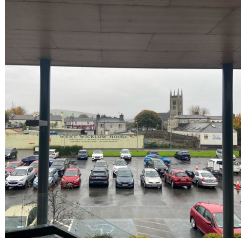
Break in development between historic town centre (background) and new Town Centre development limits integration
