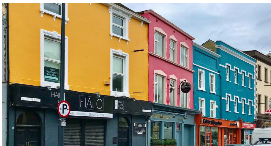
Fig.189 - Enhanced shopfronts in Dundalk
