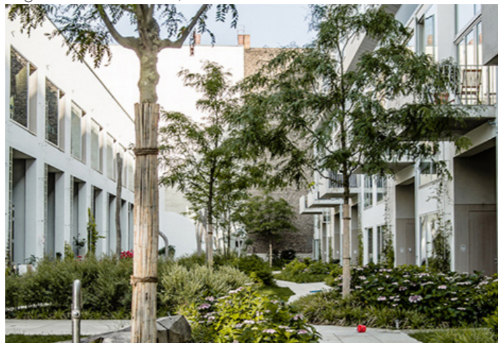
Fig.76 - BIGyard, Berlin, Germany - Zanderroth Architekten
