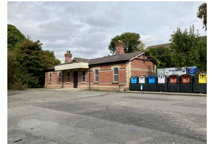
Fig.142 - View of existing train station
