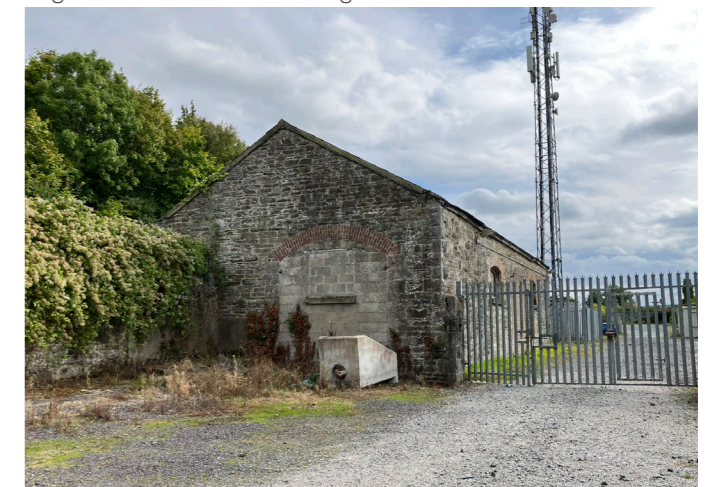
Fig.144 - View of entrance to the service yard
