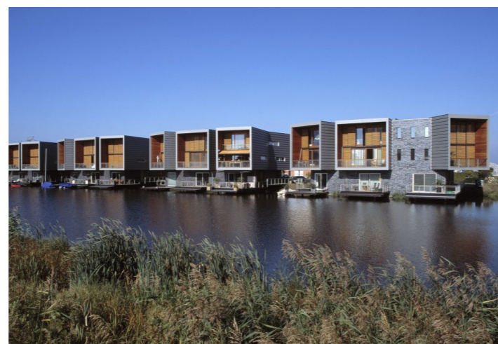
Fig.67 - Periscope Housing, Rotterdam. Joke Vos Architects
