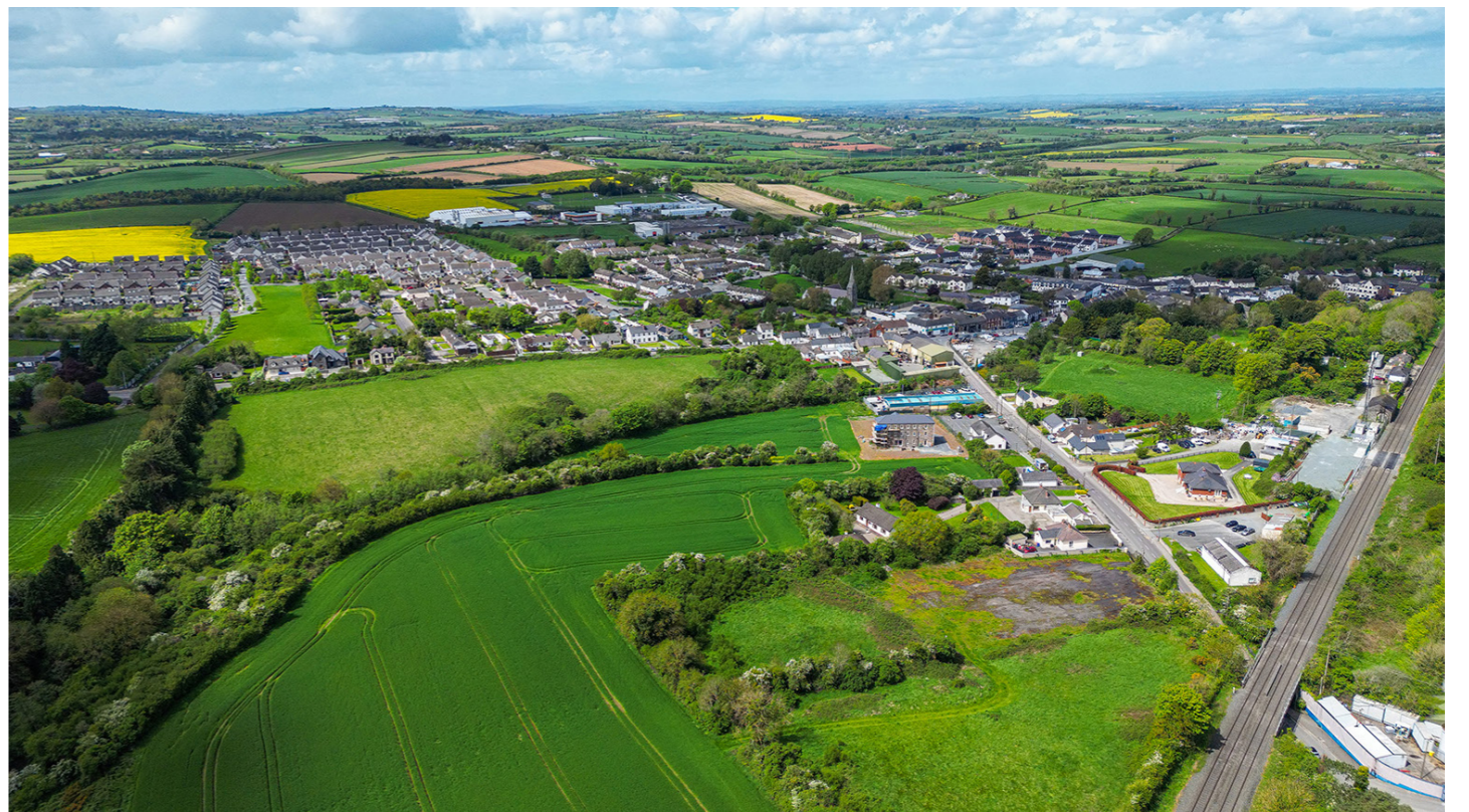
Fig.17 - Aerial views of Dunleer and its context
