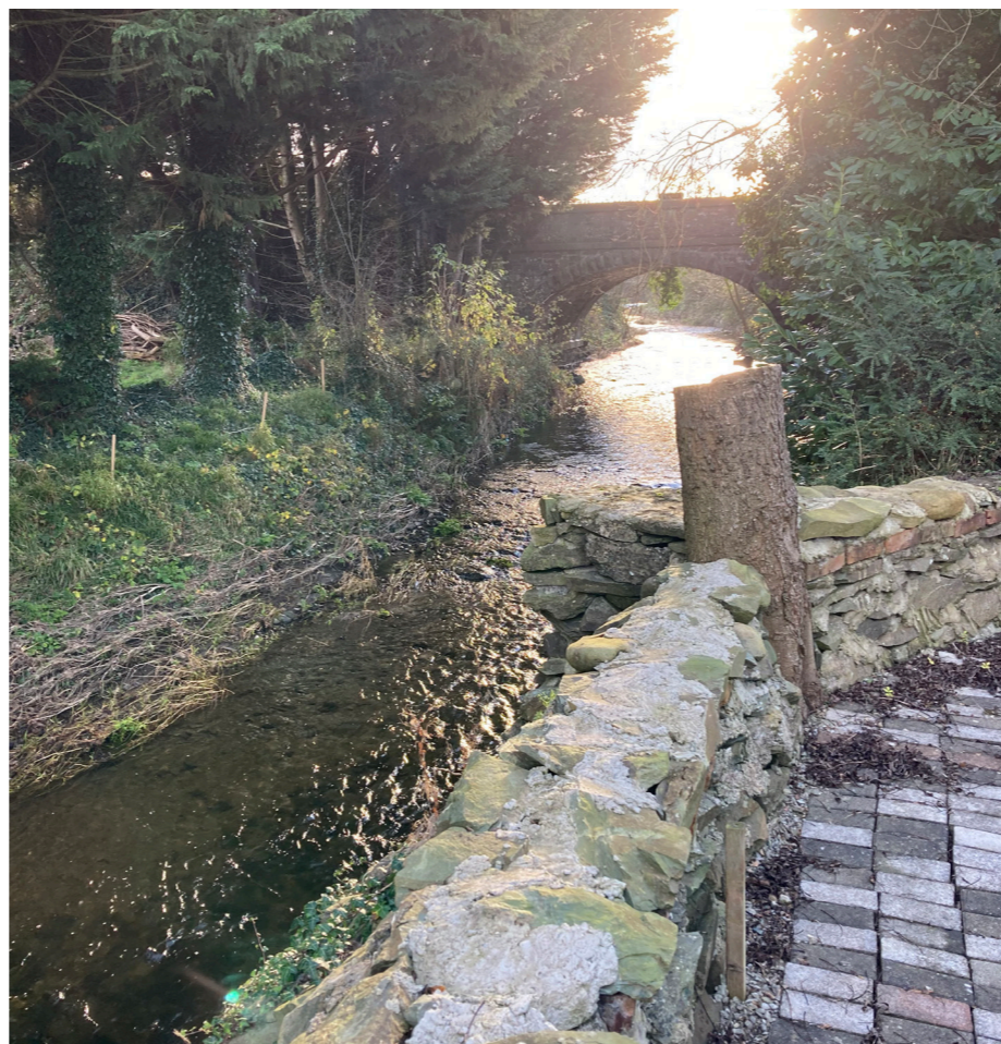
Fig.81 - White River - view of Station Road bridge
