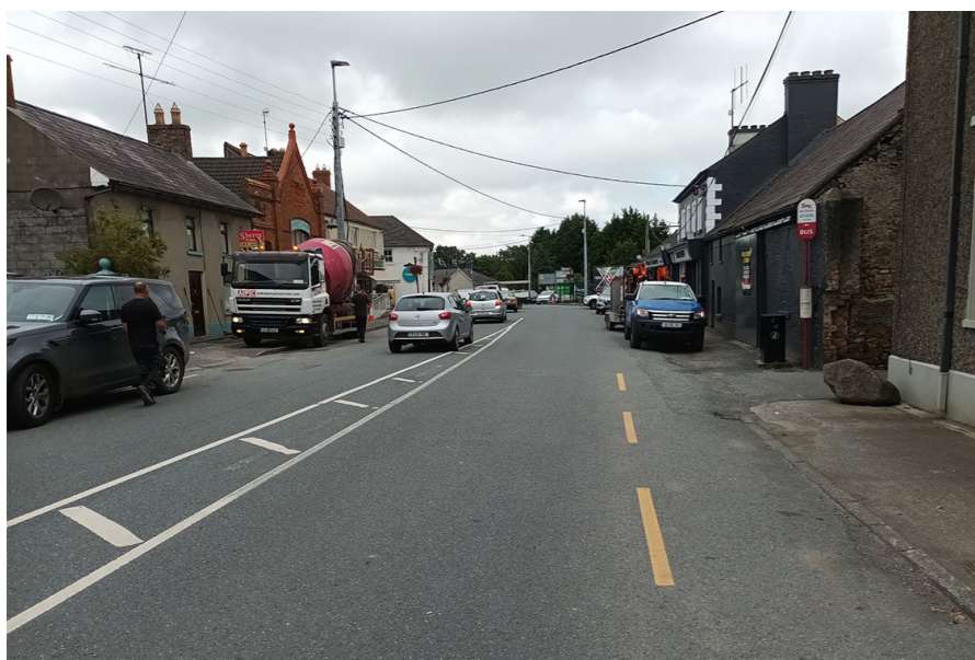
Fig.29 - Image of bus stop in Upper Main Street, highlighting the lack of seating or shelter, and the excessively narrow footway. The lack of lay-by means the bus blocks the road when stopped.
