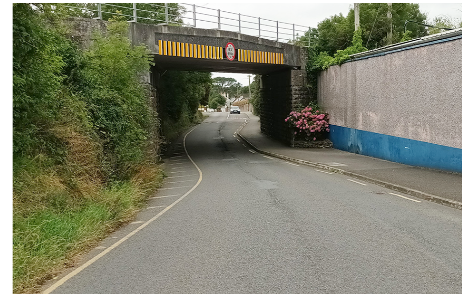
Fig.27 - Image of railway viaduct over Barn Road with narrow footway and one-way carriageway.
