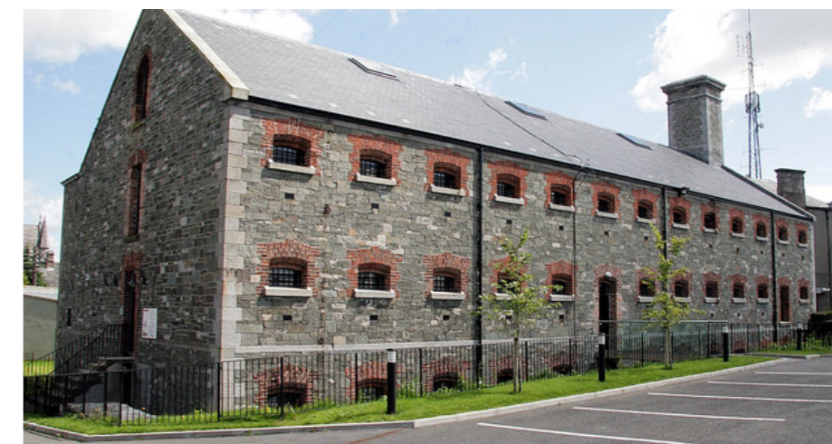
Fig.187 - Oriel Centre (former Dundalk Gaol), repair works funded by HSF.
