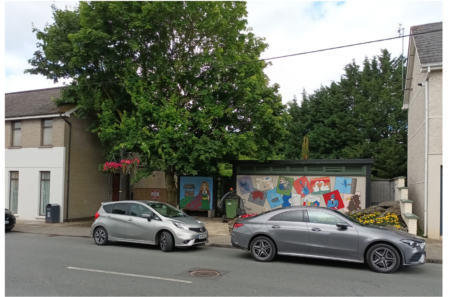
Fig.136 - View of the existing Library and public toilet block from the Main Street
