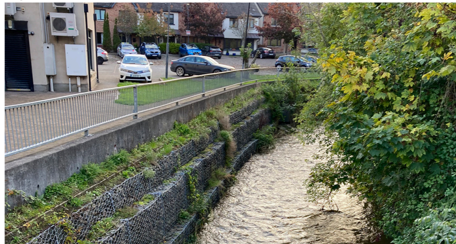
Fig.107 - Treatment of river embankment in the Forge
