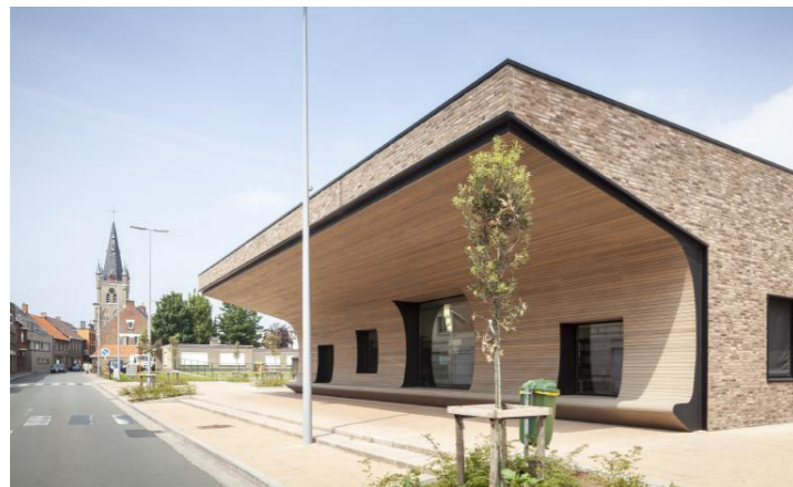
Fig.132 - Facade as public space. Cultural Centre Jonkhove, Belgium. Jozef Legrand, Dertien 12
