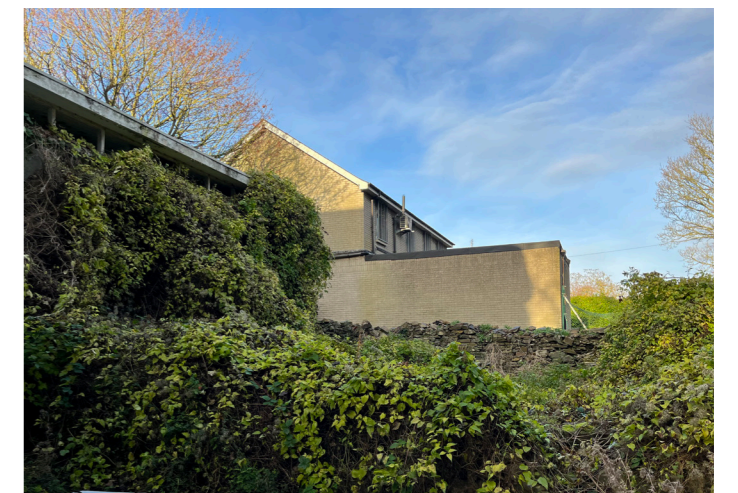
Fig.123 - Rear of former Bol building showcasing level change
