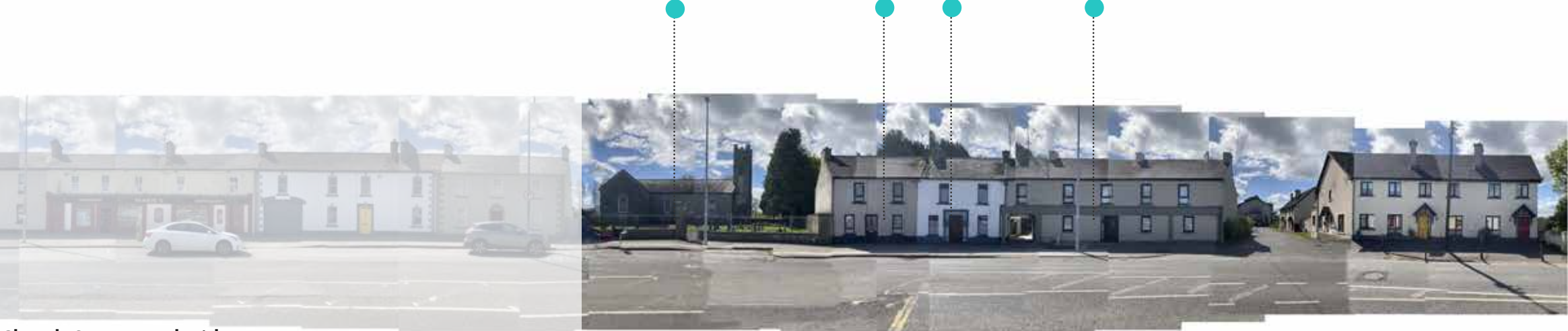
Church Street south side
