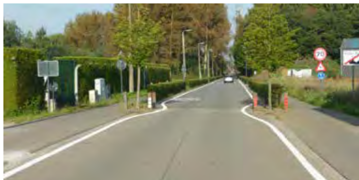
1. Traffic calming measures to reduce speed of vehicles approaching town including signage, speed bumps, and carriageway narrowing to support a lower speed environment.
