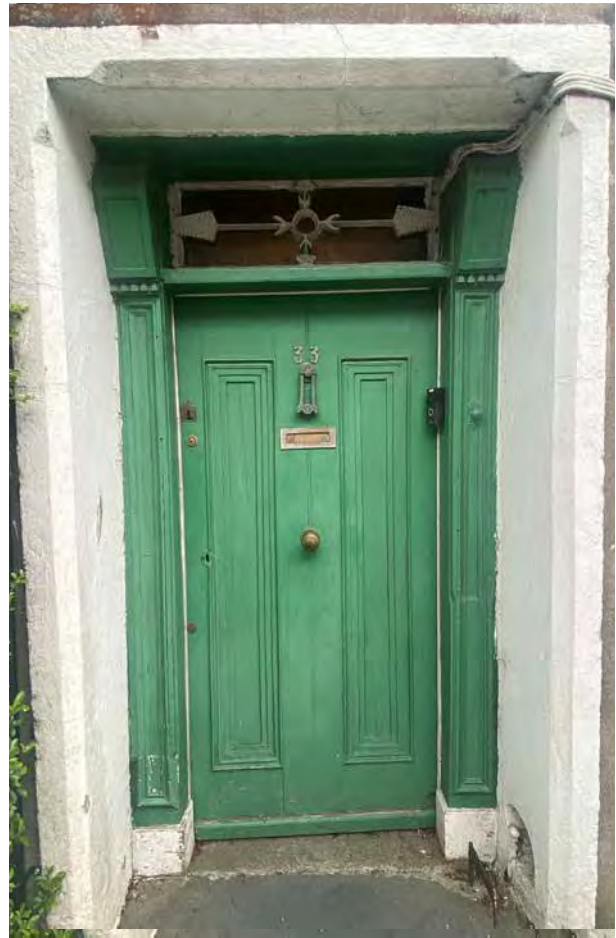
Figure 55 - Door and surround, Bridge Street
