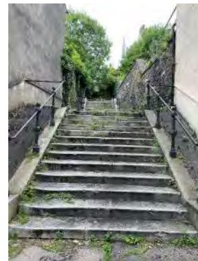
Existing condition of stairs from Mary Street to Augustinian Church
