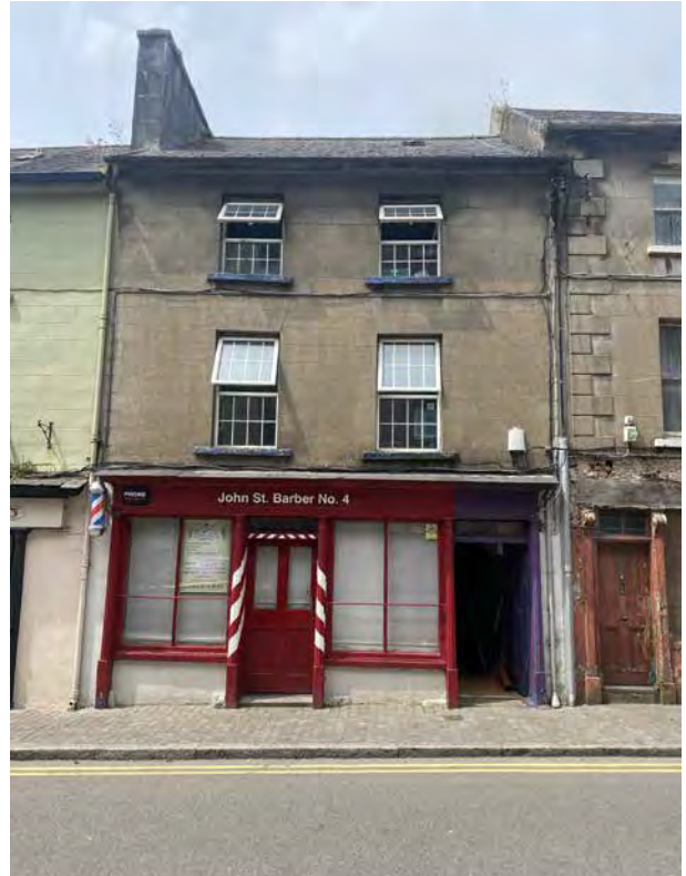
Figure 90 - Inappropriate uPVC windows, John Street
