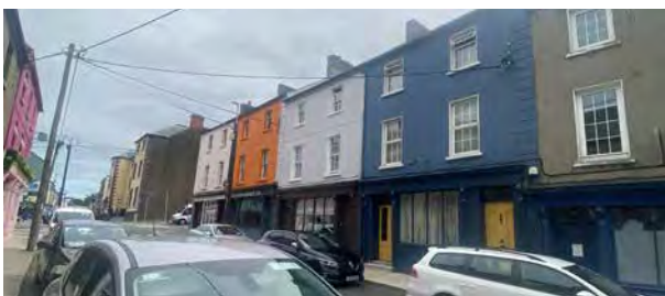
Figure 51 - Restored shopfronts, Priory Street
