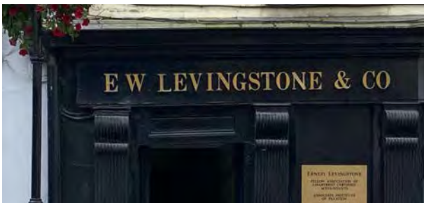
Figure 83 - Historic Shopfront: E.W. Levingstone & Co.
