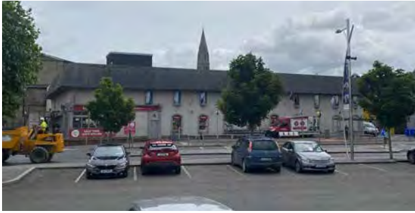
Figure 87 - Car parking and poor quality design of the SuperValu detracts from the setting of The Quay
