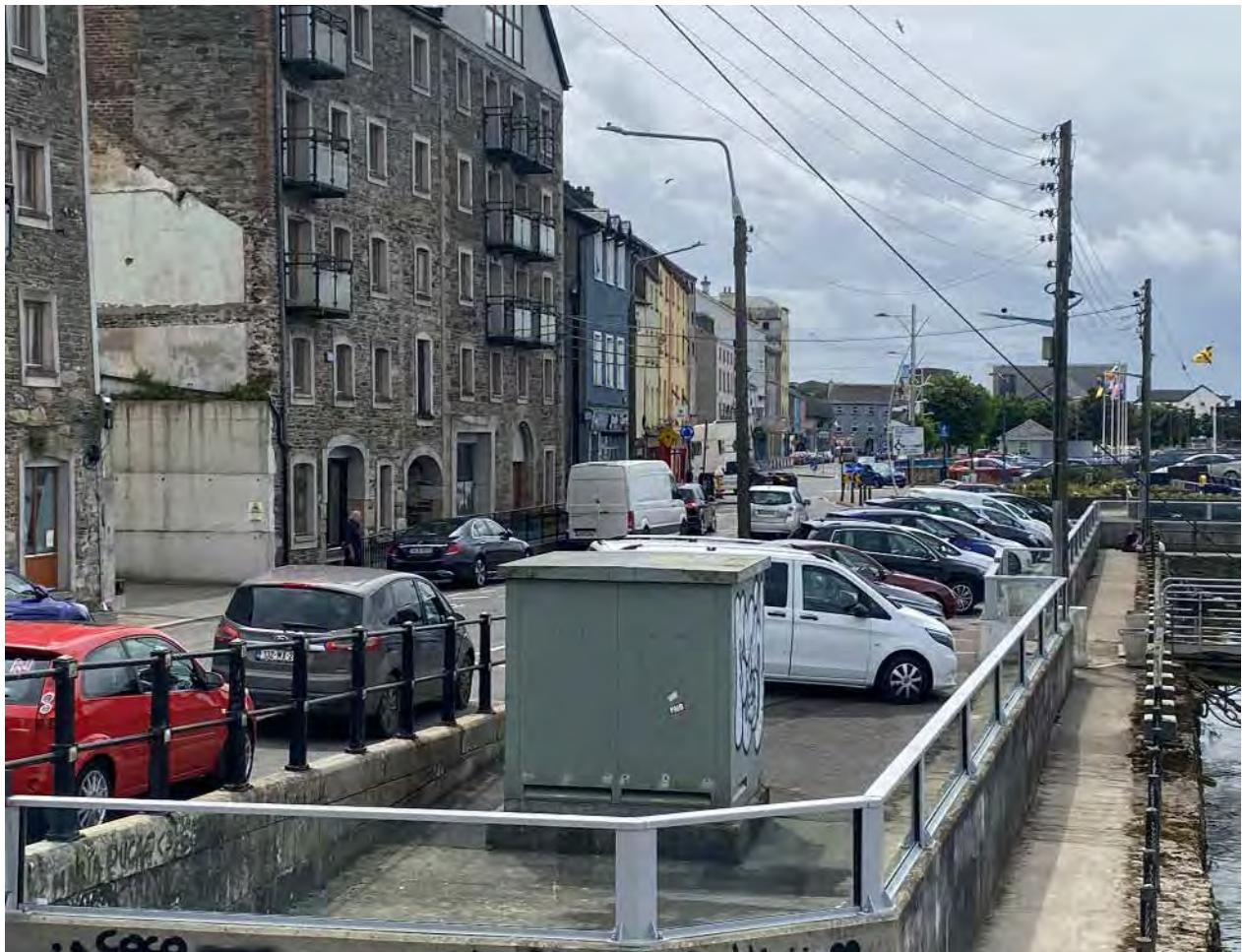
Figure 58 - Section of the historic Quay Wall visible along the Quay
