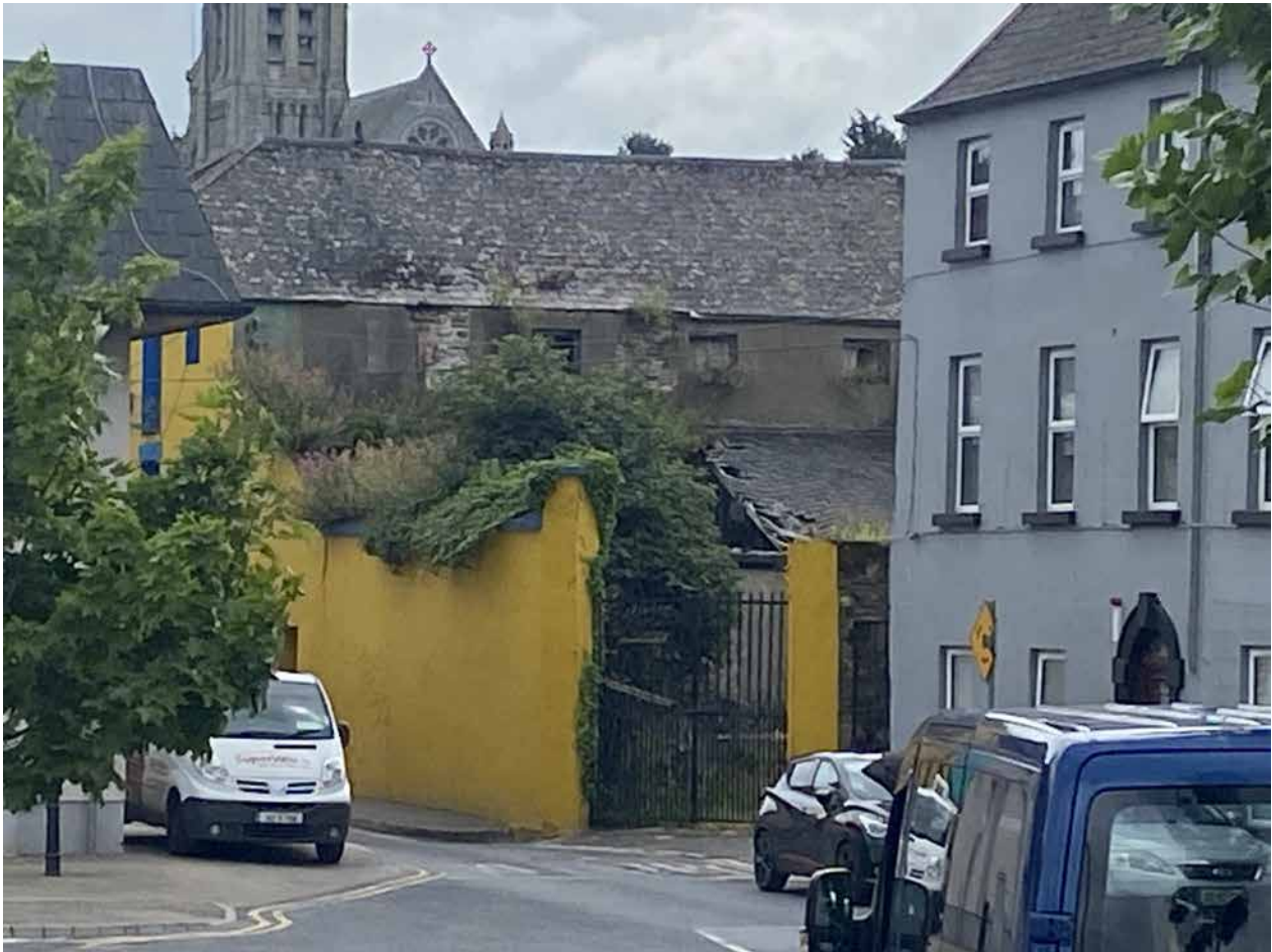
Figure 37 - Derelict site, Sugar House Lane
