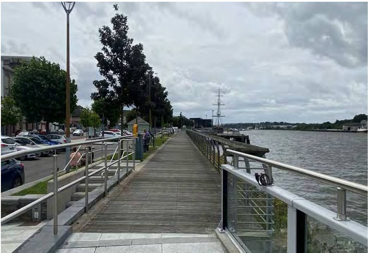
Figure 46 - View along boardwalk with historic quay wall visible to right
