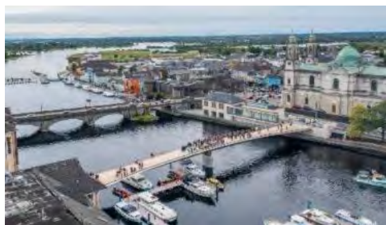
Athlone New Greenway Bridge
