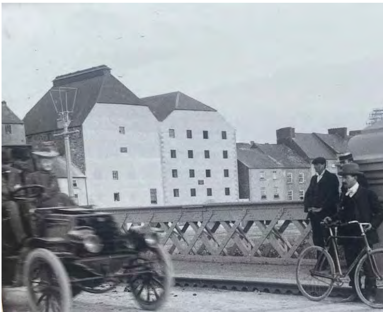
Figure 13 - Grain stores viewed from the 1869 Bridge
