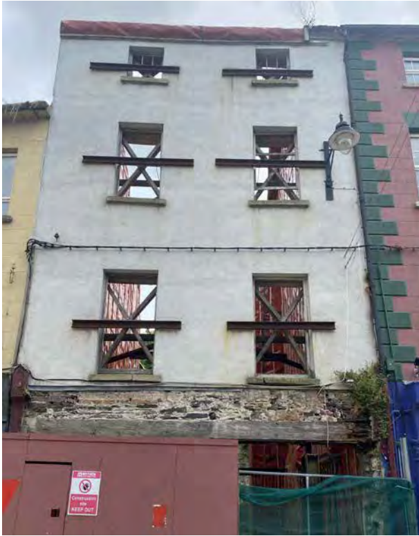
Figure 39 - Surviving facade, John Street
