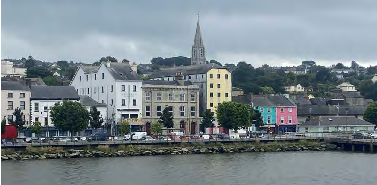
Figure 81 - View from the Bridge towards the Town
