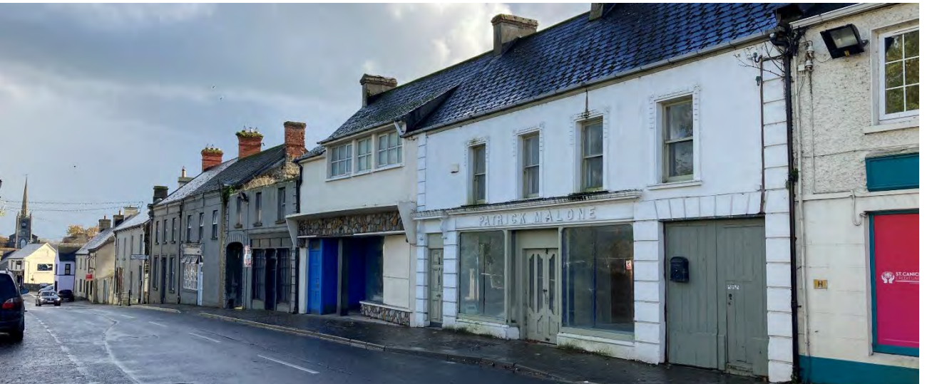
Vacant and derelict buildings along Main Street
