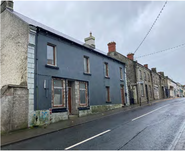
Vacant buildings / refurbishments at Main Street
