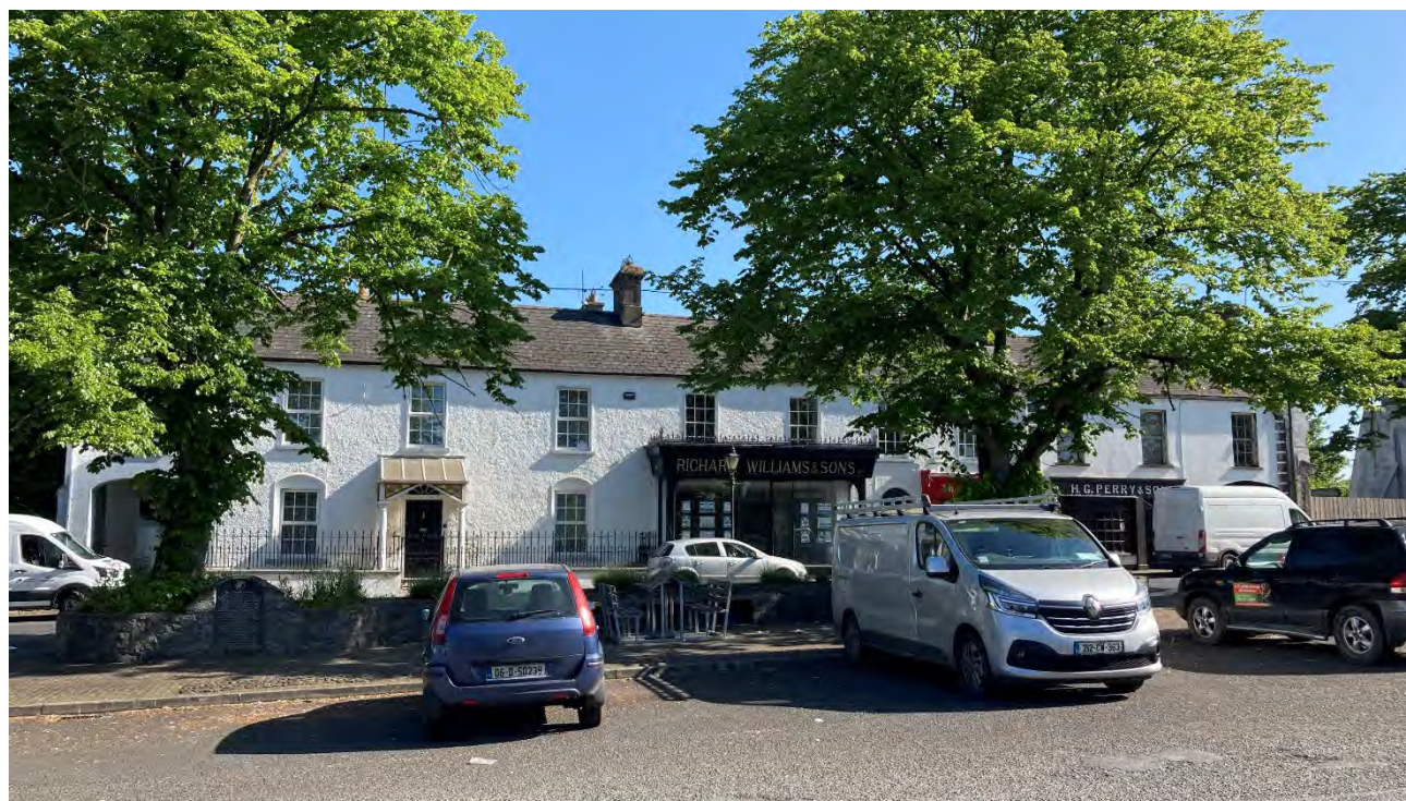
Town Square northern range of buildings
