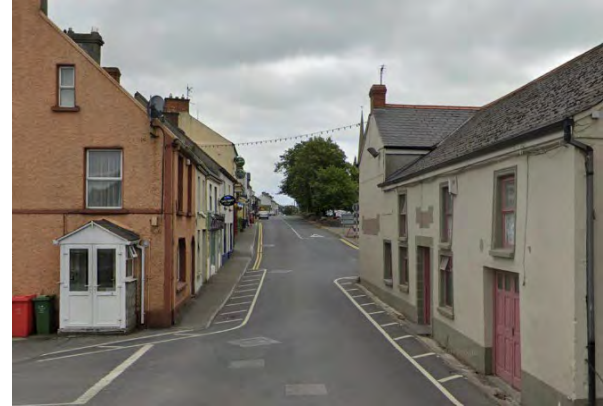
Narrow footpaths and unauthorized parking restrict pedestrian movements
