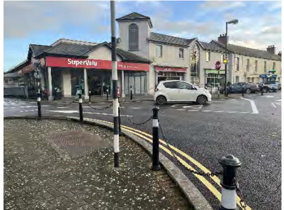
Pedestrian deterrent features
