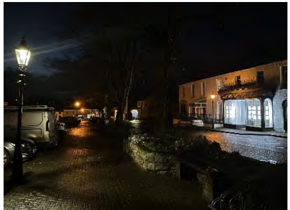
Poor quality illumination
