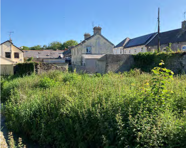
Derelict site fronting Mill Street
