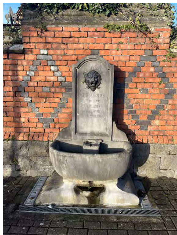
Freestanding limestone memorial fountain, c. 1920
