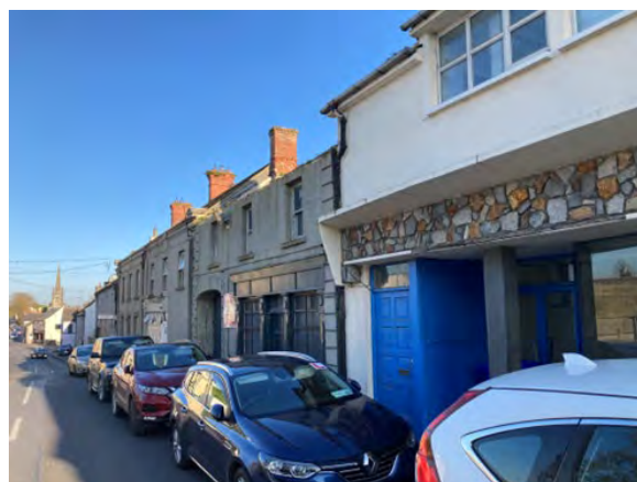
Derelict heritage building
