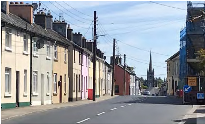
Overhead cables, Main Street
