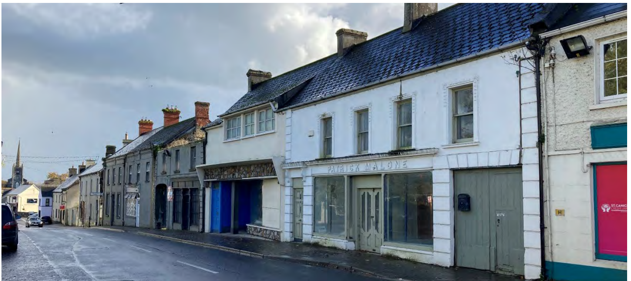
Vacant and Derelict Properties along Main Street
