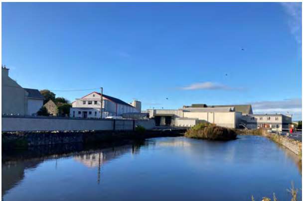
Community Centre with large boundary wall
