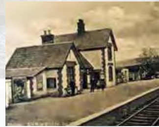
Sixmilebridge railway station built in 1859. (Sixmilebridge historical society)
