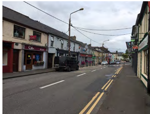
Above: Existing pedestrian environment
