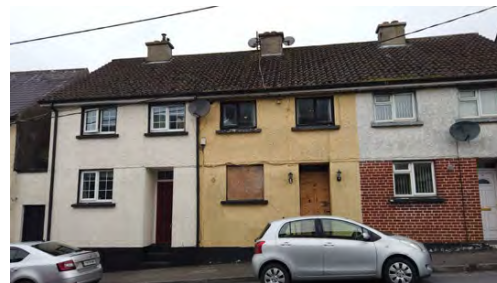
Above: Vacant residential units along Humbert Street
