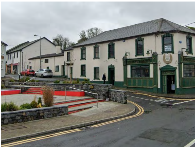
Barrier to movement at the junction of Mountain Road and Teeling Street
