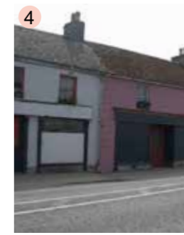
4 Traditional Shop Fronts
