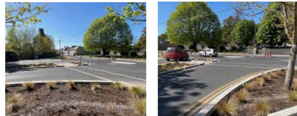
Carlow Town Raingardens
