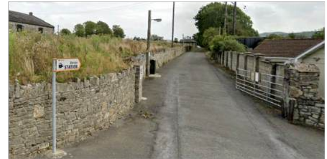
Existing access route to Rail Station
