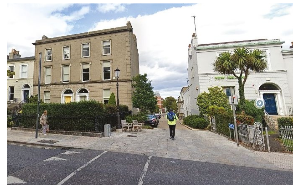
Example of retrofitting of existing junction for active travel, to improve the safety and comfort of vulnerable road users at existing priority junctions with existing path and pedestrian crossing. Note before (upper image) and after (lower image) [ Extract from 'low-cost', 'Priority Junction Tightening Measures', best practice DMURS guidance].
