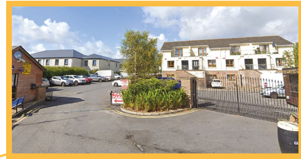
Back lot Parking, Typical
