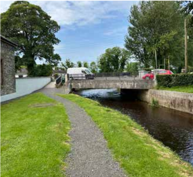
Existing river walk path and bridge at MDA buildings
