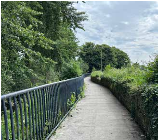
Formalised river path south of the Mountmellick Playground
