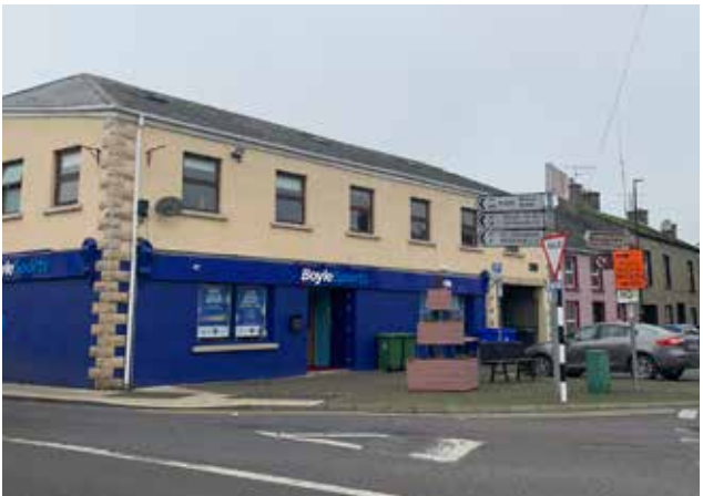
Existing junction condition at O'Moore Street
