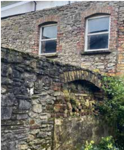
Brick and natural stone with metal work
