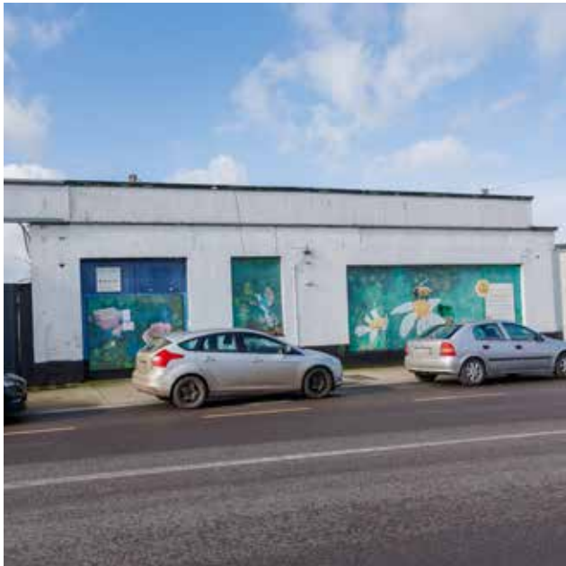
Central Garages is registered as derelict
