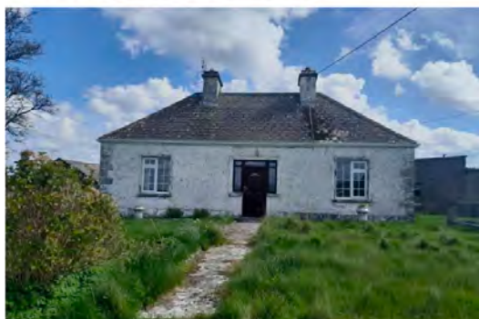
Stock picture of a derelict property
