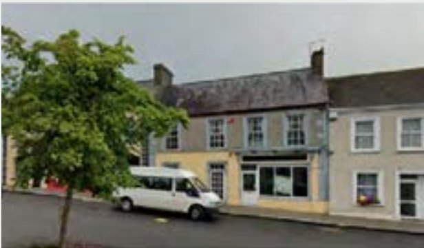
Example in Strokestown, Elphin Street Vacant - before refurbishment
