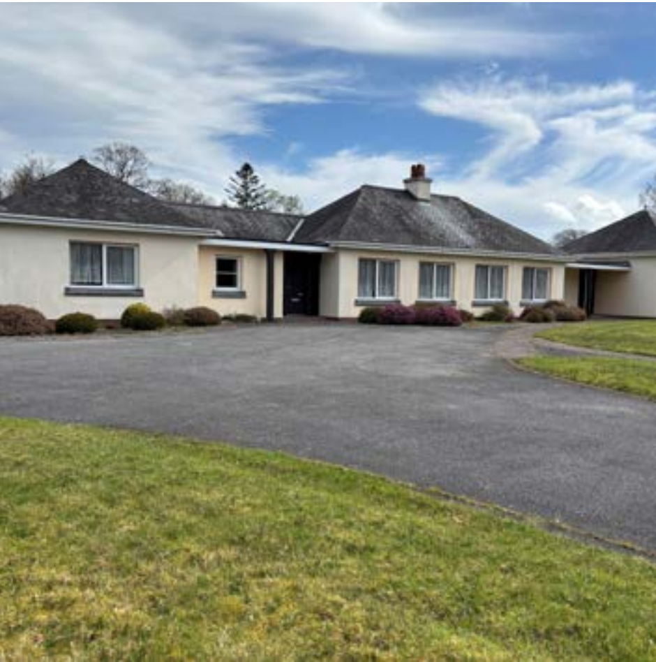
Figure 5.26: Former St. Clare’s Convent Building, Kenmare.
